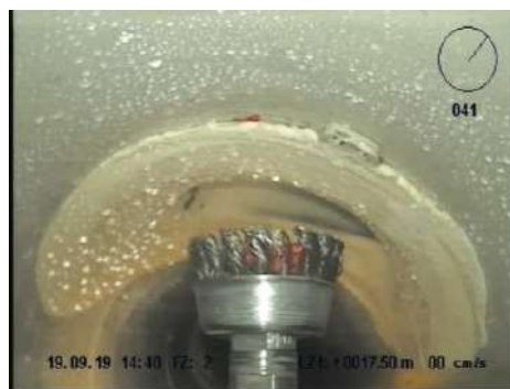
Pic.: trenchless installed house connection, ISA TOPHAT SIMONA
