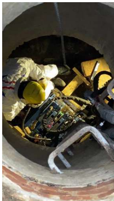
Fig.: Pulling Unit 400 KN, Tracto 400S
