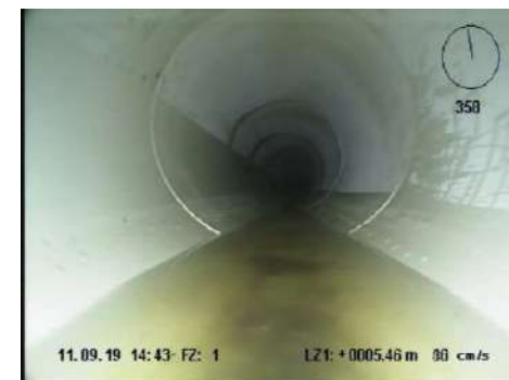
Pic.: New installed Simona Pipe
