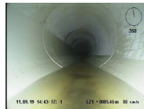
Pic.: New installed Simona Pipe
