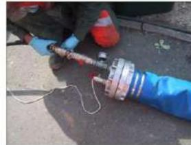
OBTURATION DE LA GAINE DE FEUTRE IMPREGNEE - MISE EN PLACE DE L'ENSEMBLE DANS LA GAINE DE PRESSION ET MAINTIEN SOUS UNE PRESSION D'AIR
