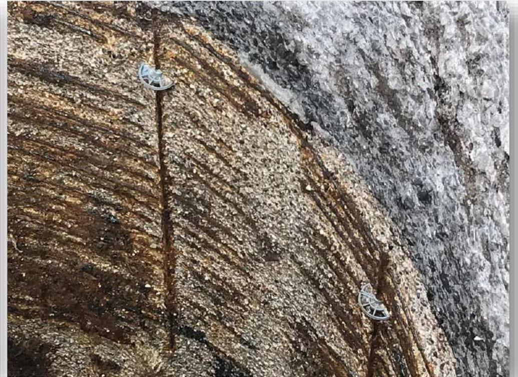
*Armatures visibles, corrosion > 5 cm*
