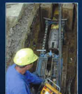
GRUNDOBURST - Eclatement - TIP - Swage lining
